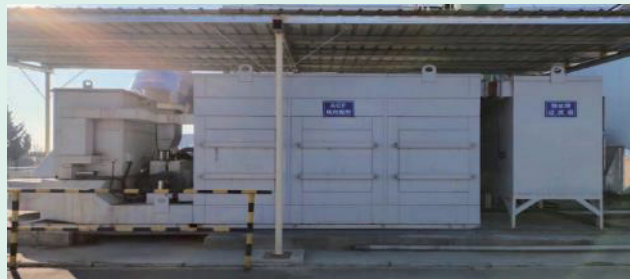
Organic Waste Gas Catalytic Combustion Purification Device 有機廢氣催化燃燒淨化裝置
